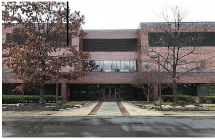
Refinancing – 300K sf Data Center Monmouth Junction, NJ
